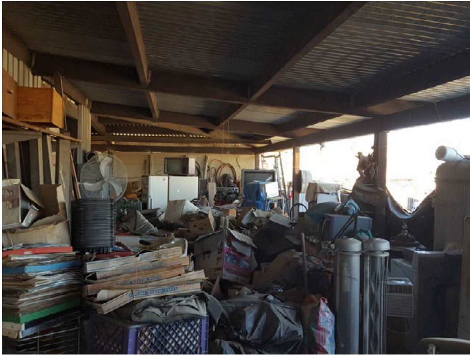
23. Enclosed areas on south side of building
