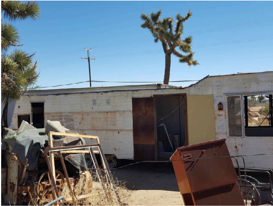
17. Trailers on northeast corner of property
